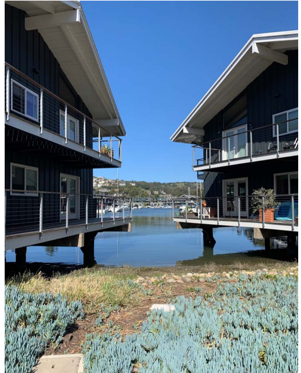
WATERFRONT HOUSING, GREENWOOD COVE AREA
